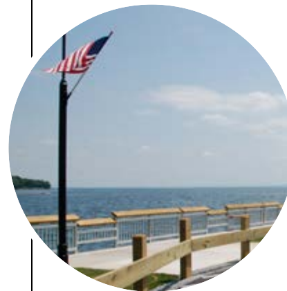
NYSDEC Dock, Cleveland NY
